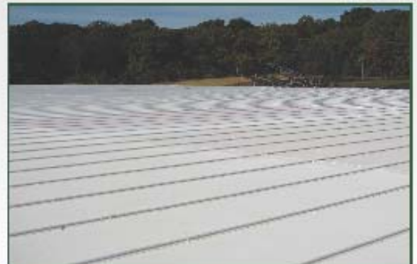
Apply 2 coats of ERSystems Acrylic 1000 Plus/SW or Polyurethane 300 Finish Coat.
