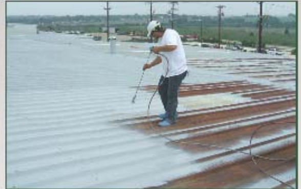
Prime all rust with ERSystems Acrylic Metal Rust Primer or Polyurethane Metal Rust Primer.
